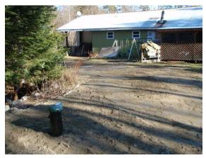
Figure 3. New bedrock supply well installed to replace impacted spring
